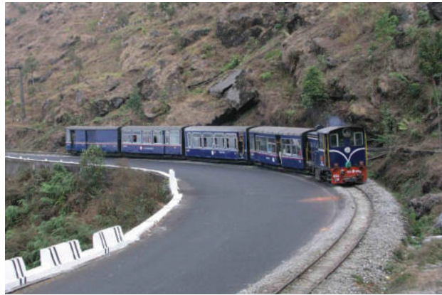
Fig.: Railway Track
